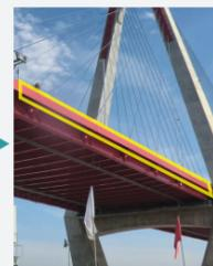
One disadvantage of cable-stayed bridges like the Nhat Tan Bridge is their vulnerability to crosswinds. This can have a negative effect on precision during construction and post-construction maintenance. In order to overcome this issue, it was initially proposed that we decrease the rectangular areas of the main girders by attaching large wind shields to their surface, but this approach was estimated to be costly given the bridge's 1.5 km span.
