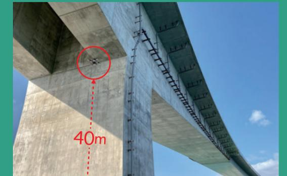
For inspections that need to be done on bridges in valleys or with high piers, the use of a drone can sometimes be cheaper than more conventional methods like the use of large inspection machines or rope access. The autonomous drone will face the bridge and fly alongside it, capturing comprehensive images that the operator can use to assess the extent and spread of damage. In Japan, everything down to the delivery of inspection results has been digitally automated.
